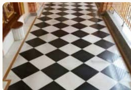
Marble Flooring Works
